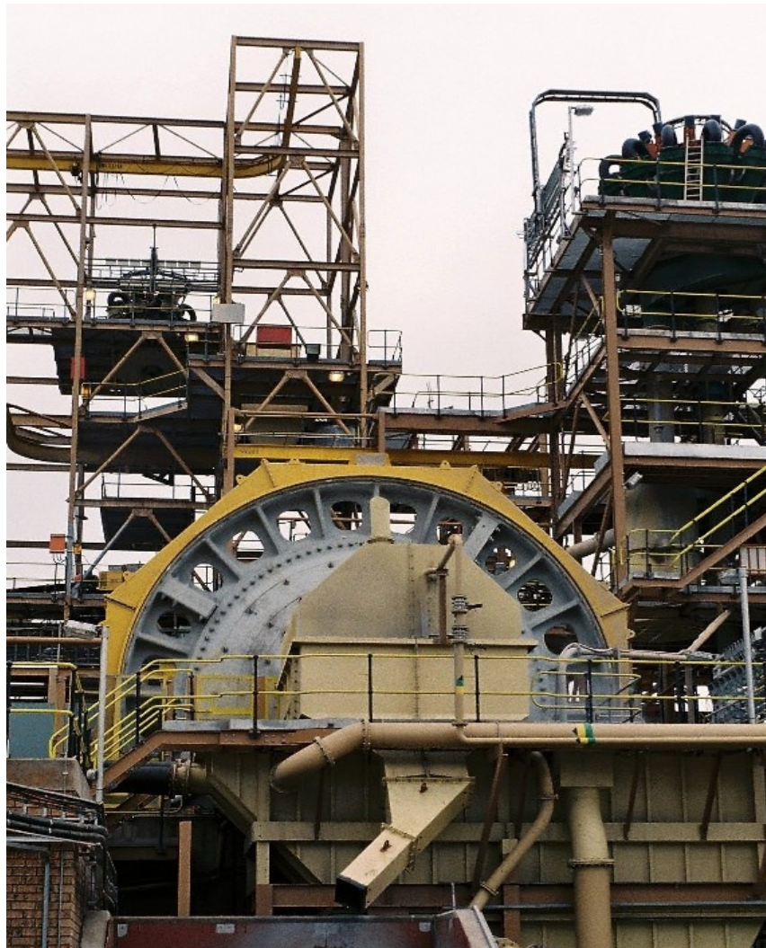
A base metal crusher unit in Mpumalanga
